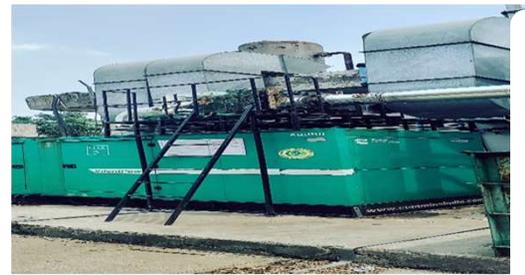
**Retrofit Emission Control Device Installation for All DG Sets**
